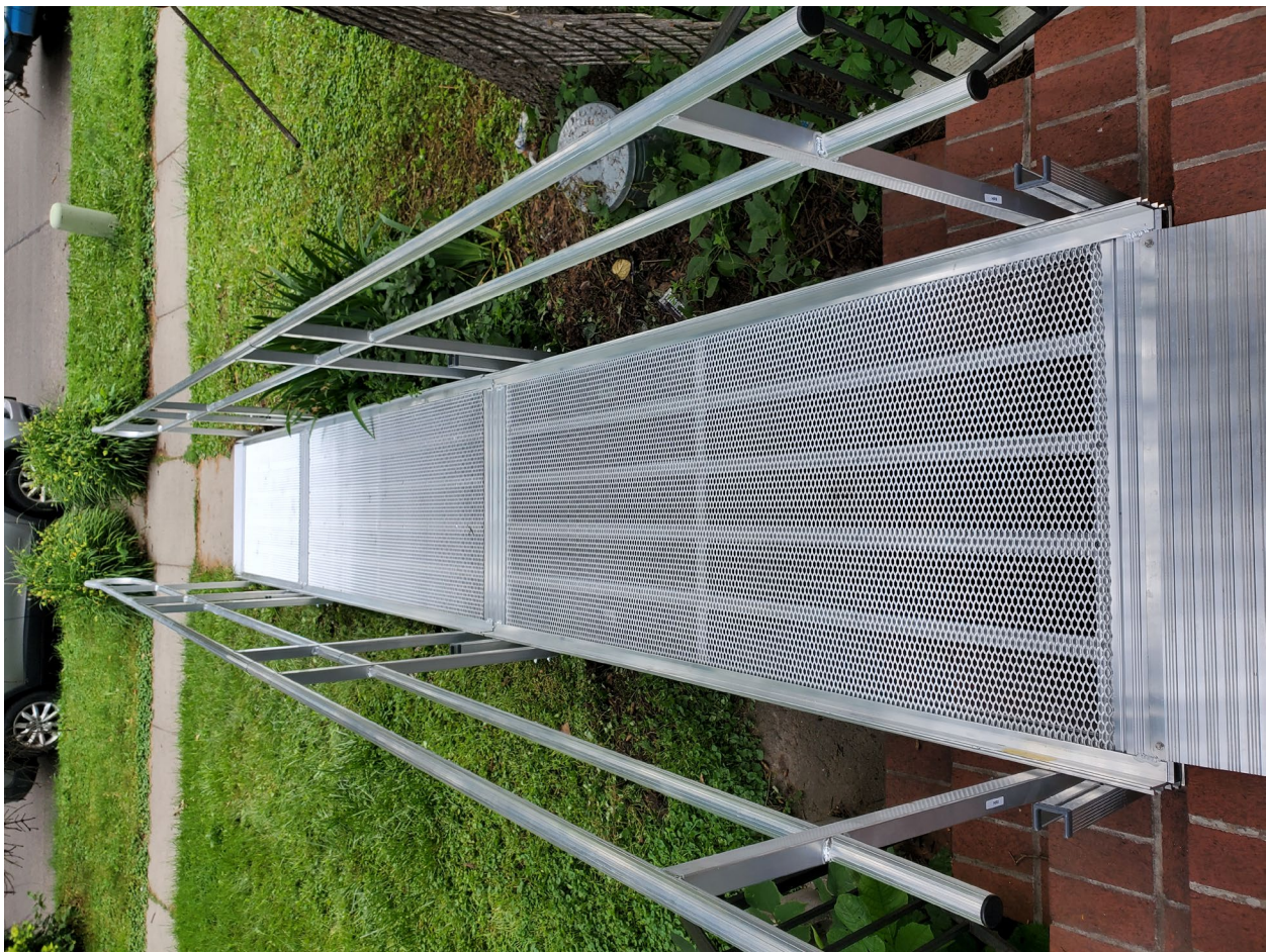
Installed aluminum ramp
