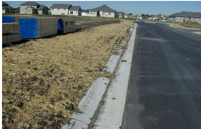
Boulevard recently seeded with disk anchored straw mulch applied to prevent sediments from entering the curb line.
