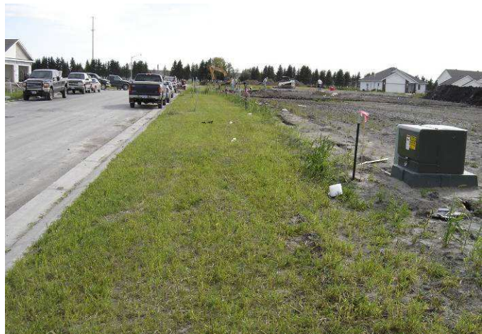
Established grass buffer strip. These should be left undisturbed until the final lot grading and sodding or seeding.
