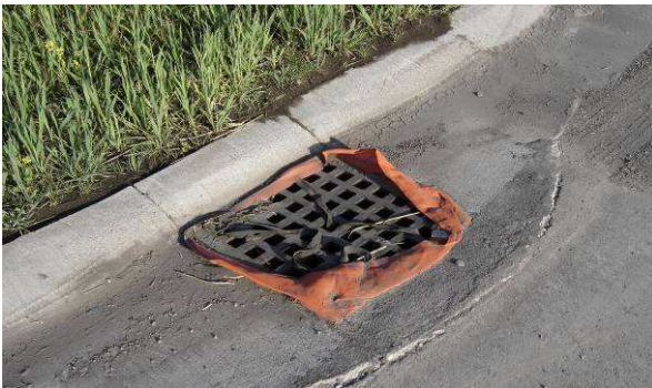
Inlet protection installed in a new subdivision. Their purpose is to capture any sediments that are in the curb line while still allowing stormwater to drain.
