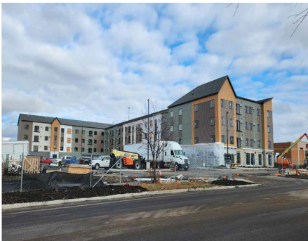
Phase II Compass Apartments
